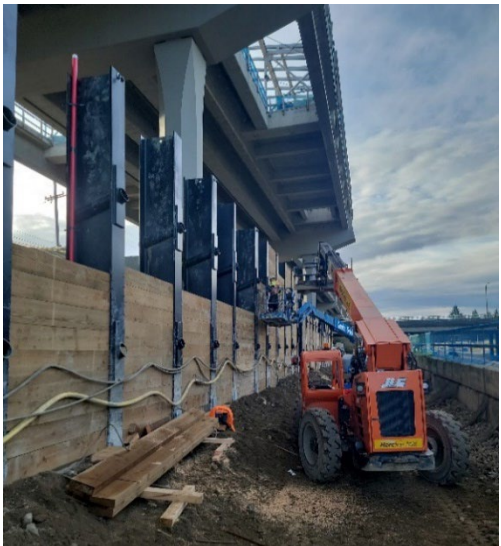
A soldier pile retaining wall will support the station plaza.
